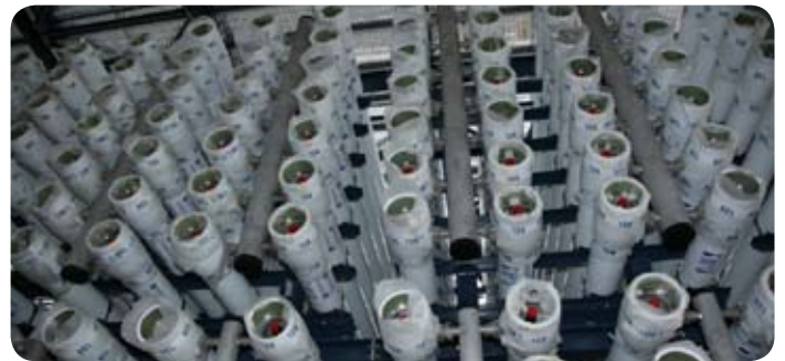
Membranes used at desalination plants as part of the reverse osmosis procedure.
